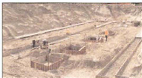
April 2002 Phase 1 Footprint of Fire station
