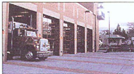
January 2003 Fire Station Complete
