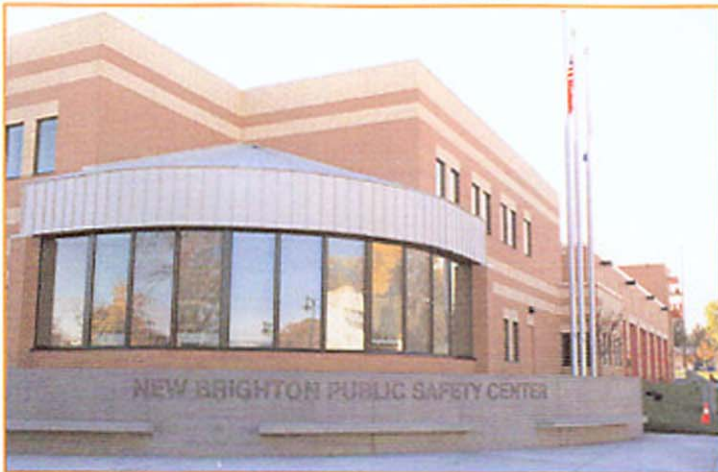
September 2003 - Completed New Brighton Public Safety Building
